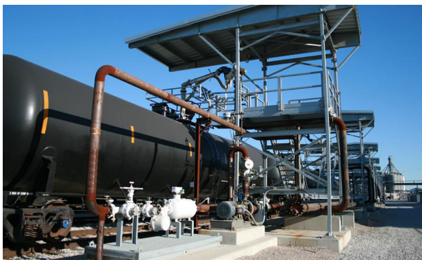
Rail Loading Terminal
